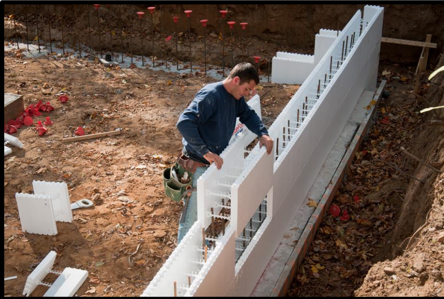
AN INSULATED CONCRETE FORM (ICF) HOUSE IS CONSTRUCTED OF HOLLOW FOAM BLOCKS THAT SNAP TOGETHER LIKE LEGOS, AND THEN ARE FILLED WITH CONCRETE.
